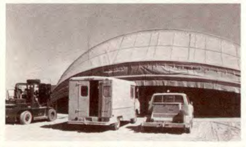
Portable hangars like this can be set up in hours. They provide shelter from the desert sun and protection from sandstorms while working on aircraft.
